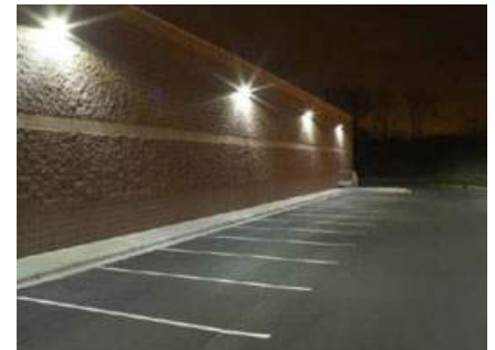
RWP LED in Use
